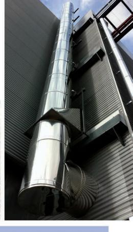
Besides the factory made metal exhaust systems the jeremias group produces frestanding and widshields chimneys for big electric power generators.
